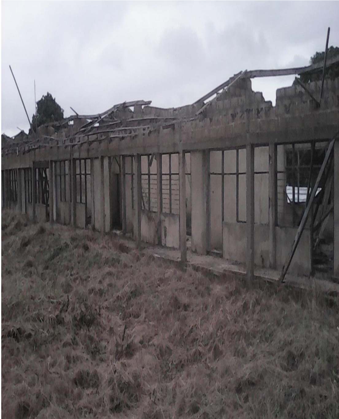
Fig.2.5: Wasted materials on classroom block Author's field note 2015
